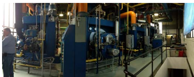
FIGURE 2.10: North Heating Plant
