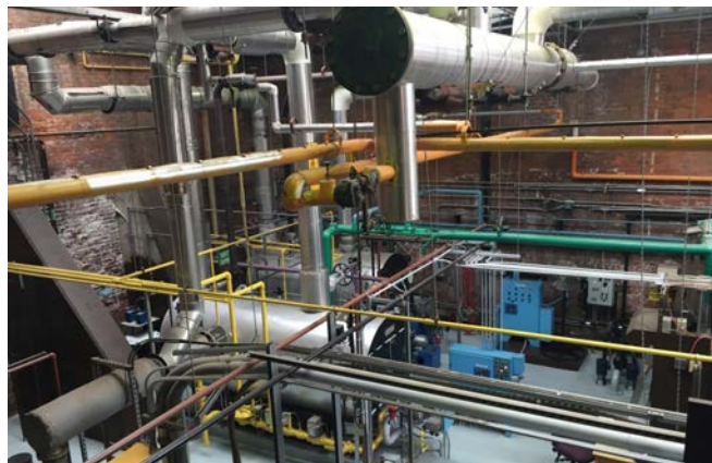
FIGURE 2.9: South heating Plant
