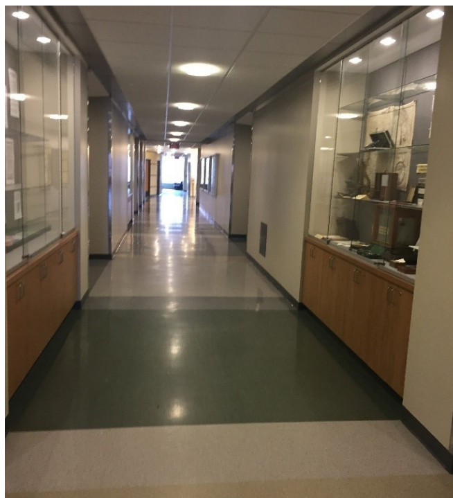
FIGURE 2.12: Eastern Interior Lighting
