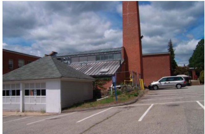
FIGURE 3.1: Eastern Heating Plant
