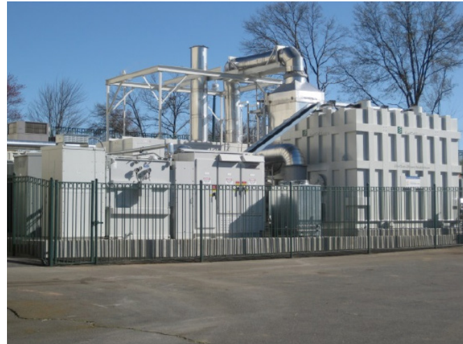
FIGURE 2.12: Central's Fuel Cell System
