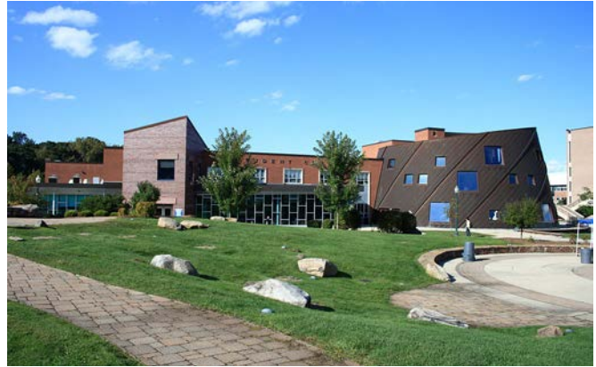
FIGURE 1.1: Central Connecticut State University Student Center
