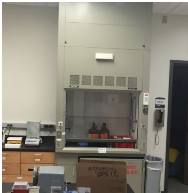
FIGURE 2.11: Science Building Fume Hood
