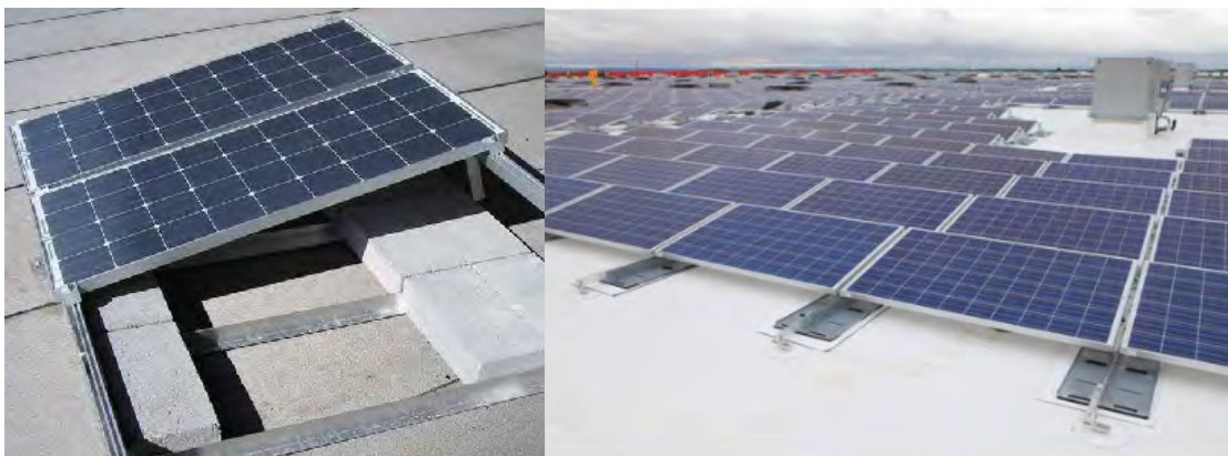
FIGURE 2: Ballasted and Fastened Solar PV
