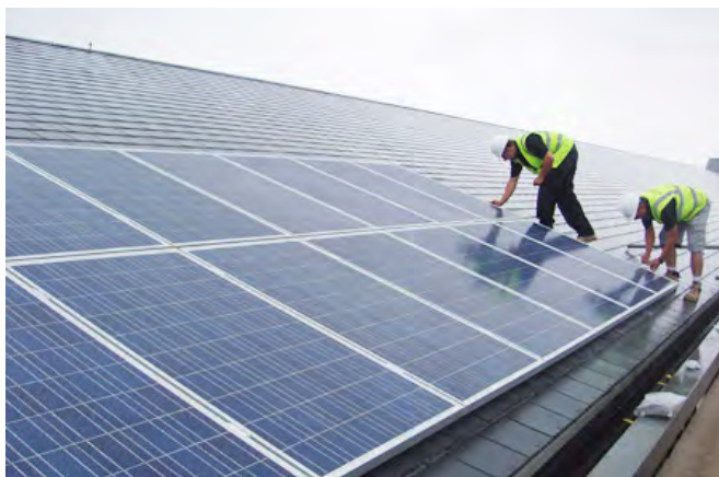
FIGURE 5.2: Solar Photovoltaic (PV) Installation
