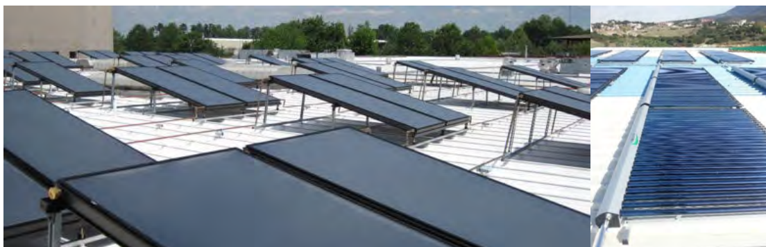
FIGURE 7: Flat Plate and Evacuated Tube Solar Thermal Collectors
