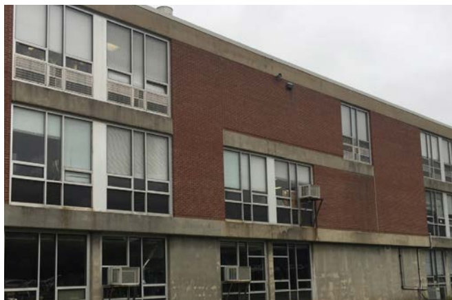
FIGURE 2.5: North Haven Campus Air Conditioning
