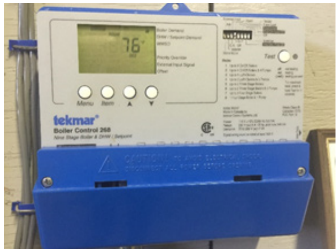
FIGURE 2.2: Boiler Control System
