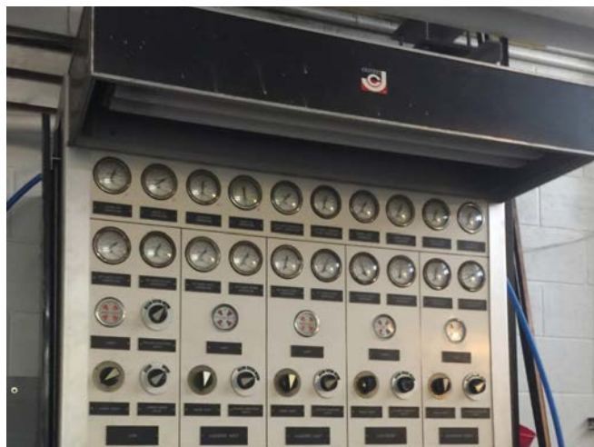
FIGURE 2.6: North Haven Heating Control
