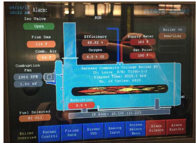
FIGURE 2.4: Boiler System Monitor
