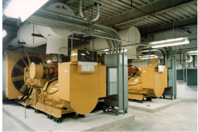
FIGURE 3.1: Emergency Generators
