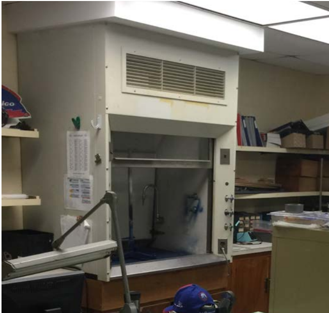
FIGURE 2.8: North Haven Fume Hood
